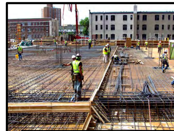
Over 300 miles of rebar would stretch from Minneapolis to Green Bay.
