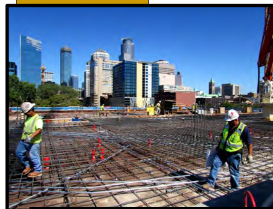
Coordination of rebar installation with mechanical and electrical embeds
